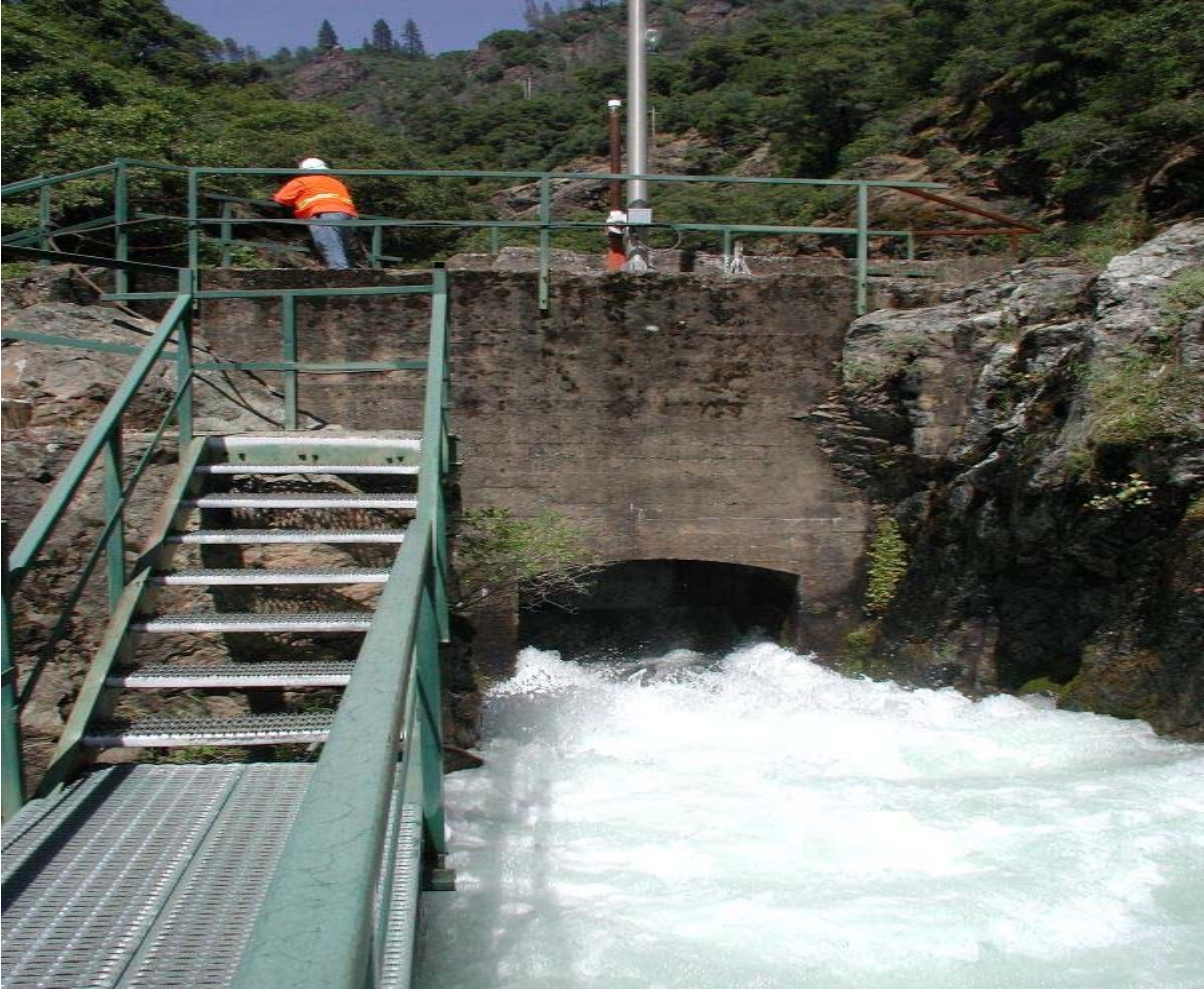
Figure 4. Lower Centerville Canal immediately downstream of the headworks sluice gate.
