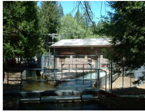
Figure 1.1.1-8. Toadtown Powerhouse Ground View
