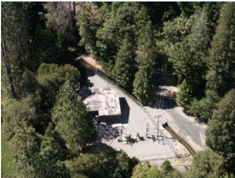
Figure 1.1.1-7. Toadtown Powerhouse Aerial View
