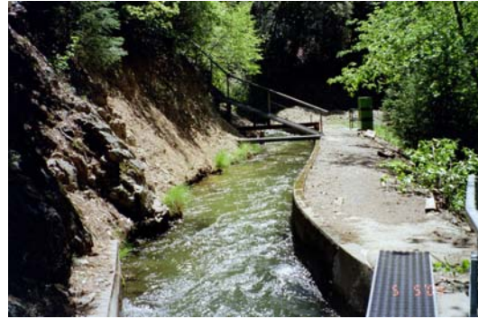
Figure 1.1.2-2. Butte Creek Canal
