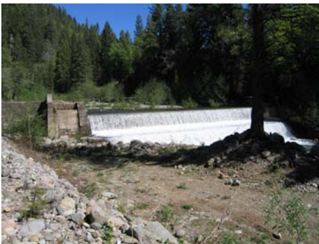
Figure 1.1.1-5. Hendricks Head Dam
